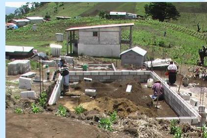
Reconstruction in process in Guatemala
